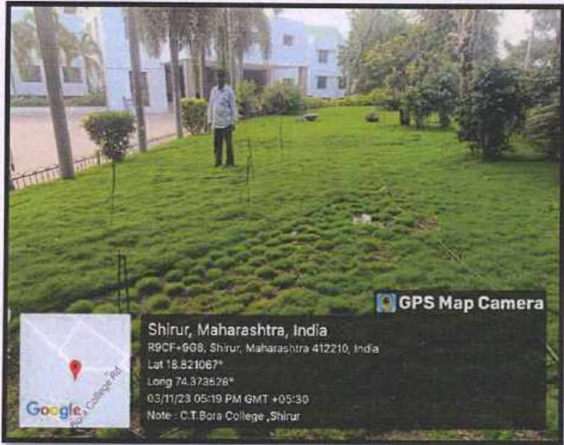
* Photograph of Water Sprinkler System in the garden
