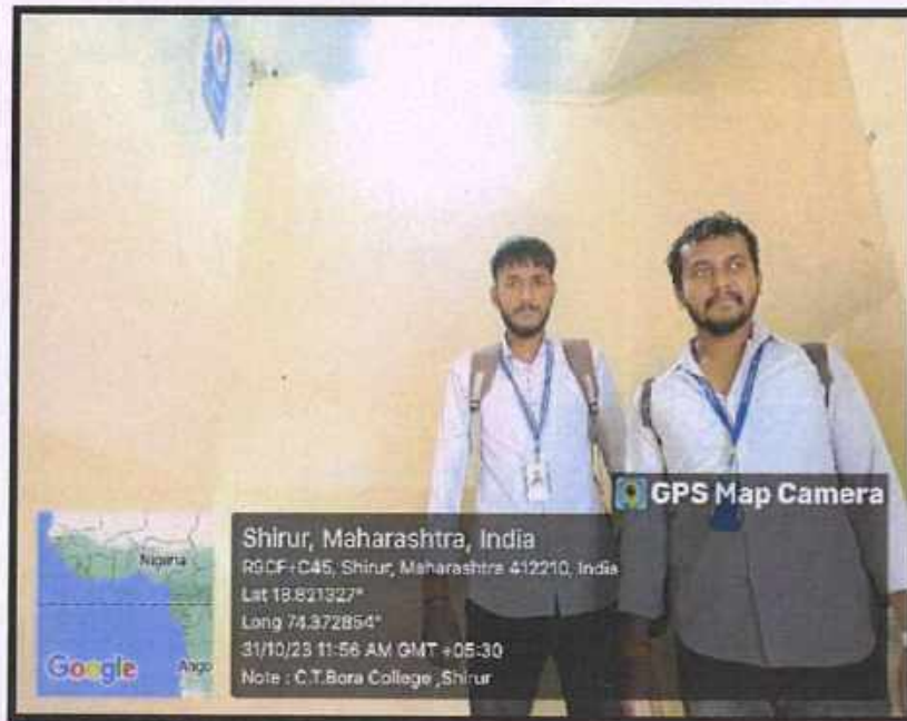
* Photograph of Sensor based LED bulb on the Staircase of Library
